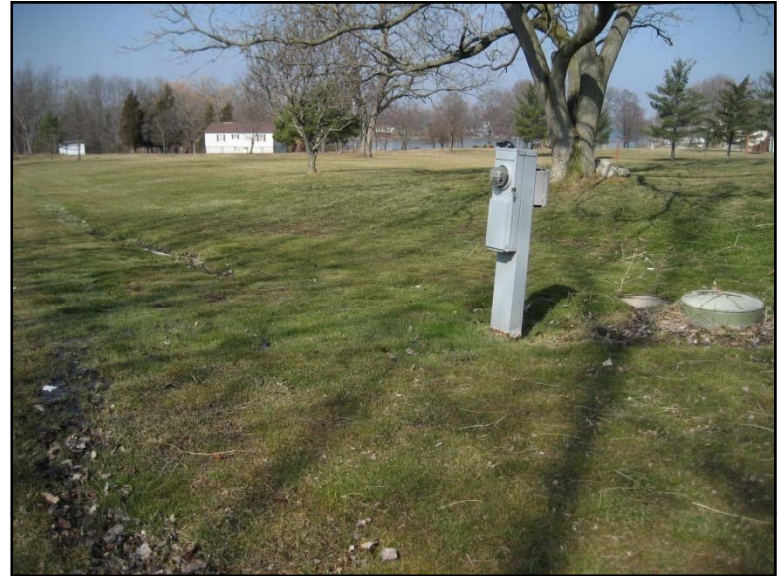
Photograph 2: Electric meter and grinder pump on the northern property boundary.
